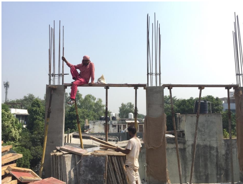
Fig 5. Shuttering for slab casting, Saxena, 2023
