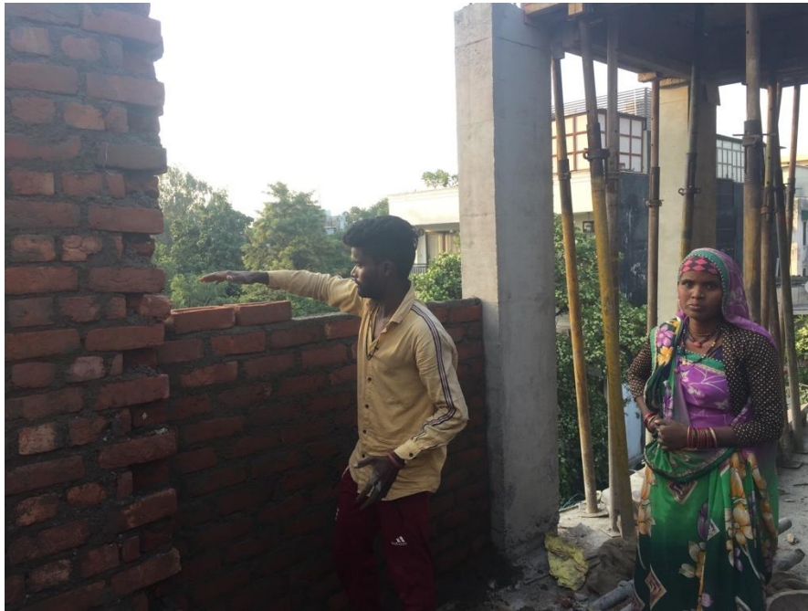
Fig 6. Brick laying by Mistry with helper(wife), Saxena, 2023
